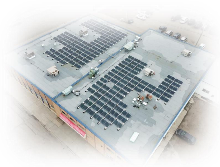
Mannawanis Friendship Centre aerial view of new roof with solar panels reinstalled.
